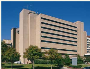
U. T. M.D. Anderson Cancer Center at Houston R. Lee Clark Clinic Building
